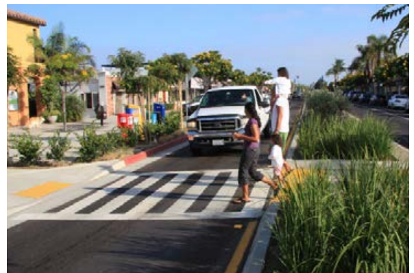
Above (Right): The roundabout on La Jolla Blvd in San Diego, CA has reduced crossing distances from 64 feet to 14 feet. Pedestrians no longer have to cross multiple high-speed lanes at once.
