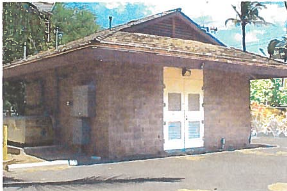
A typical liquid waste pump station in Kihei
