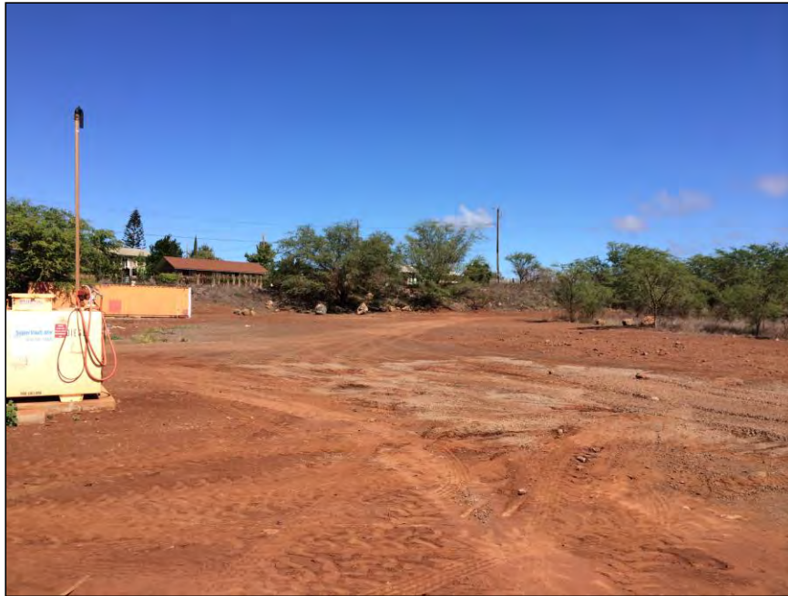
Photo 12: Overview of the Ohukai Access Road – TMK: 2-2-002: 016.
