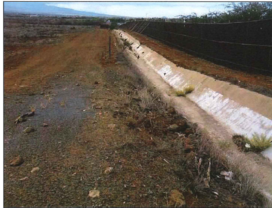
View of concrete drainage culvert that runs along the western boundary of the subject property and under Piilani Highway.
