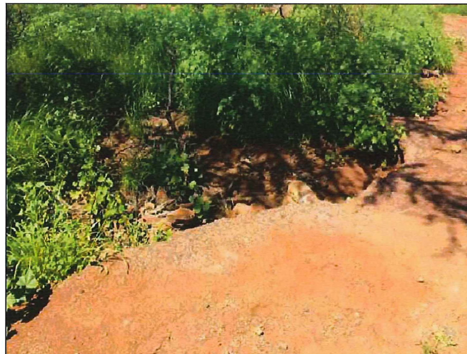
View of Drainageway "A" located on the property.
